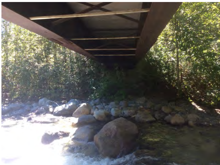
Right Bank Abutment when facing downstream
