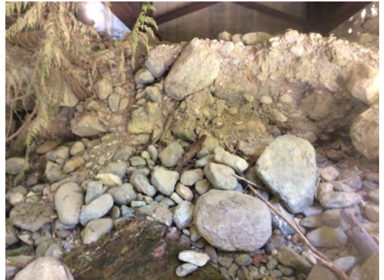
Left Bank Abutment when facing downstream
