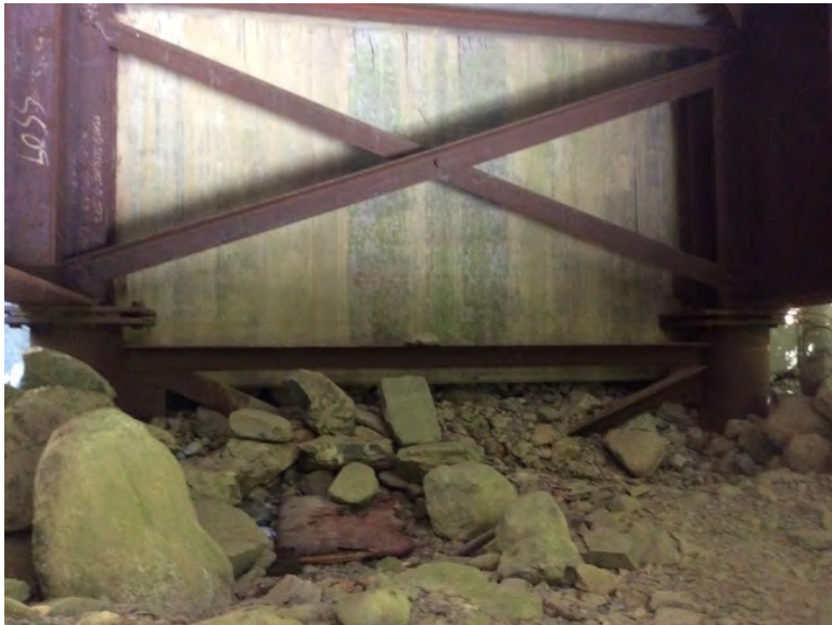
Left Bank Abutment when facing downstream
